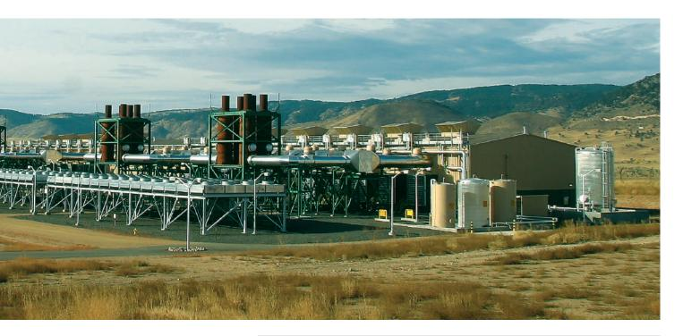
**Fig. 1.** Plains End power station in Colorado. This facility with a combined output of 231  $MW_e$  is an example of a modern gas-fired commercial power plant based on gas engines. It has been in operation since 2001 (section I) and 2006 (section II), providing a way to balance unstable wind power output.
