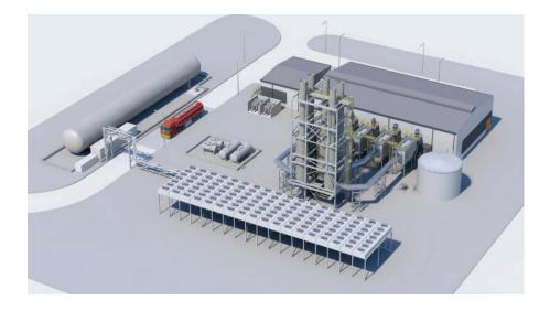
**Fig. 14.** Visualization of a 50 MW gas engine power plant with a 500 m<sup>3</sup> (17,700 ft<sup>3</sup>) LNG storage system visible on the left-hand side. This tank would be sufficient for 24 hours of continuous plant operation at full load. The gas may be supplied in liquefied form by trucks, ships or railroad, depending on the local infrastructure.
