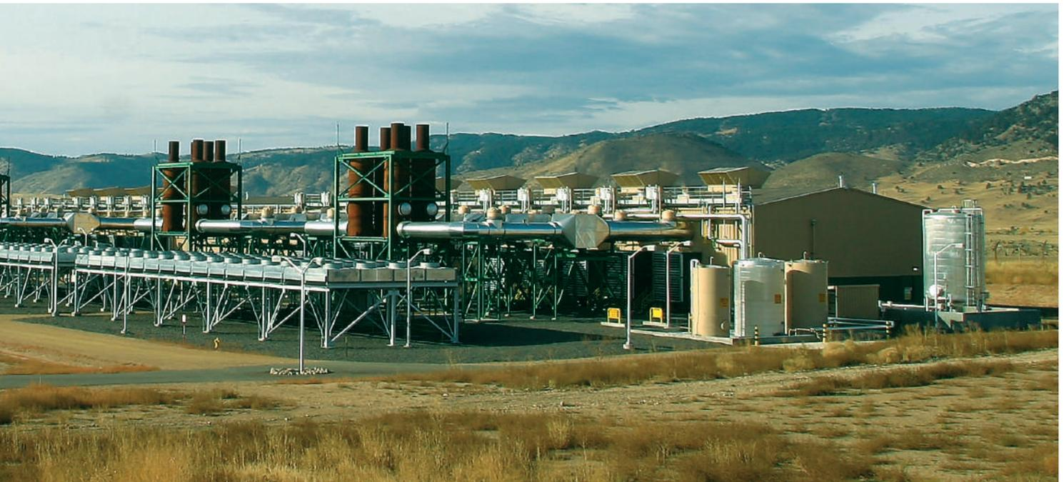
**Fig. 1.** Plains End power station in Colorado. This facility with a combined output of 231 MW<sub>e</sub> is an example of a modern gas-fired commercial power plant based on gas engines. It has been in operation since 2001 (section I) and 2006 (section II), providing a way to balance unstable wind power output.
